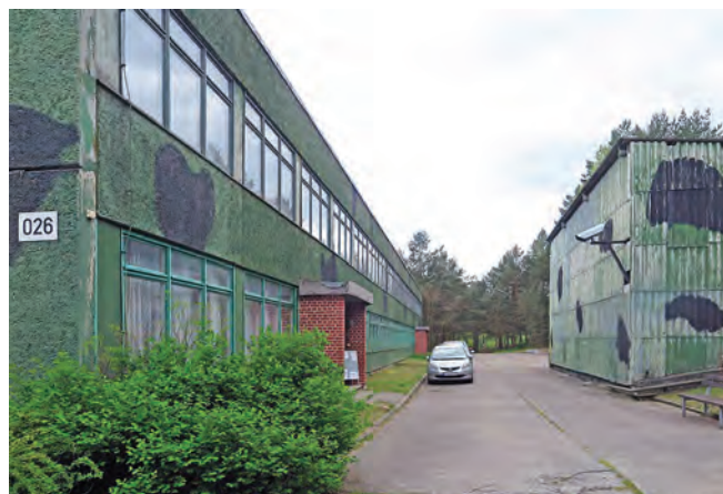
The Harnekop main building, just your average office block, though with a bigger than average basement.
